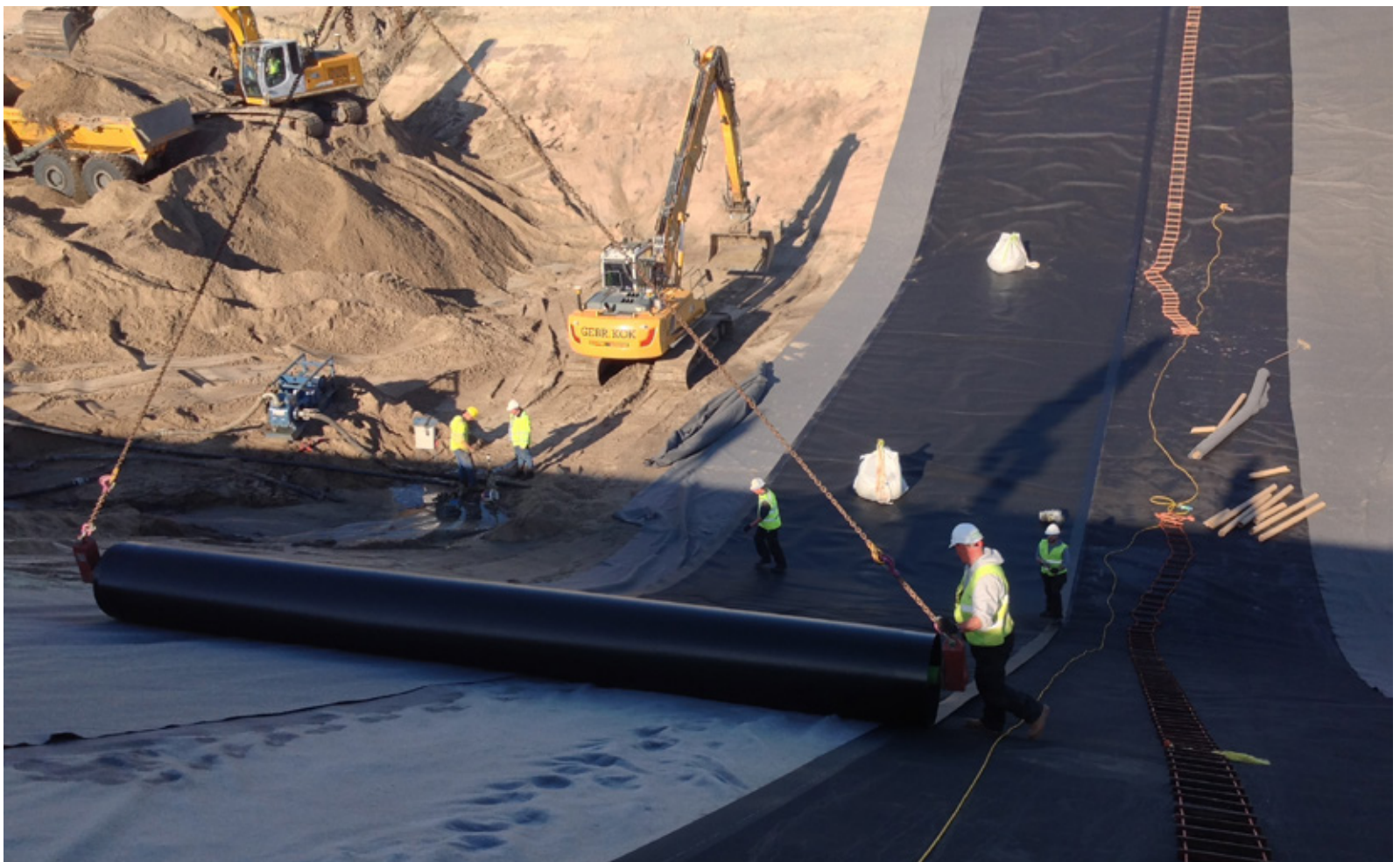
Figure 5 - Example of proper installation using a protective non-woven geotextile at the subsoil and topside of the geomembrane, working sequence with excavation works and installing method at large slopes [Gerritsen]
