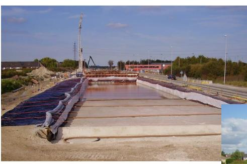
Installation with winches to each side building pit, submerging geomembrane
